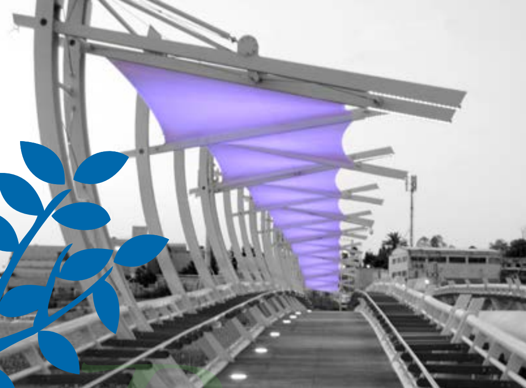
Pipes Bridge at Be'er Sheva River Park
